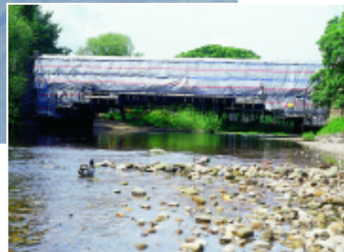
Bridge maintenance and the associated traffic management measures.
