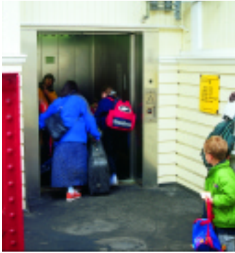
Rail stations are becoming more accessible by various means eg, via the provision of lifts such as at Halifax Station.
